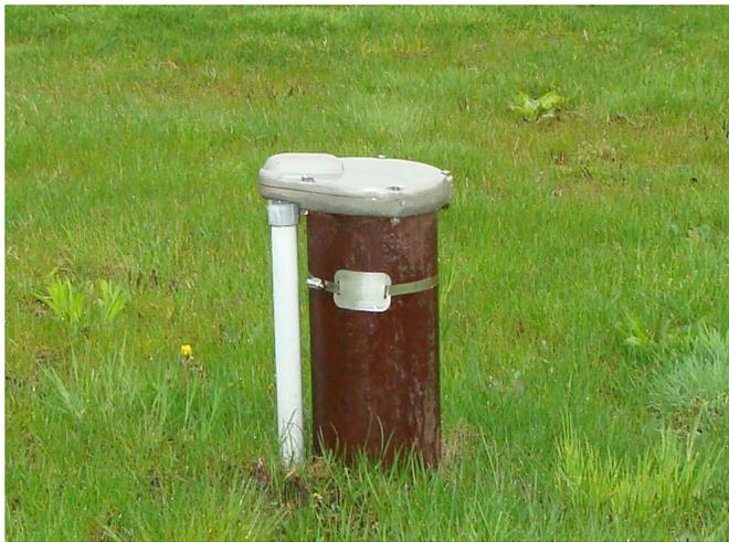
*Properly constructed drilled well shown with a vented and vermin proof well cap, electrical conduit for submerged pump (to left of well casing), identification tag (linked to Water Well Record), casing extends at least 40 cm above the ground, and ground that is mounded away from well casing.*
