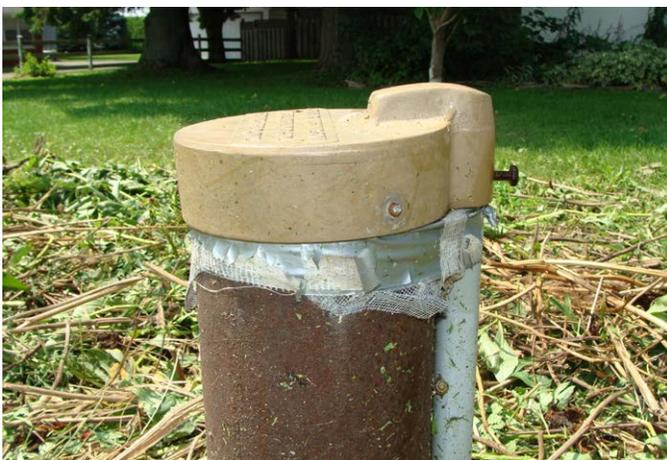
*An inadequate well cap may allow pests and other types of contamination to enter into the well, and may not allow for proper ventilation.*
