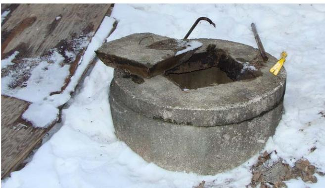
*It is important to regularly inspect and maintain your well and test the water. This is a drilled well located in a pit (these are no longer allowed to be constructed). If you have a well located in a pit, you could upgrade it so that the well casing extends at least 40 cm above the ground. NEVER ENTER A PIT.*
