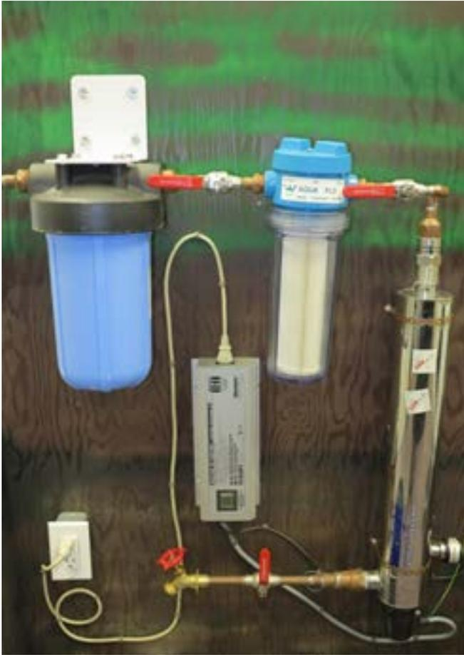
*An example of a filter and ultraviolet disinfection system.*
