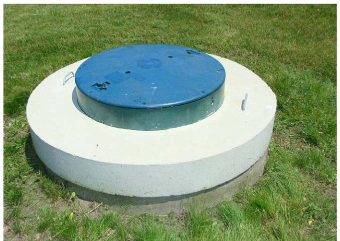
*A dug well with an upgraded sturdy lid (that is properly vented and vermin proof) reduces the amount of contamination that can enter the well. Older wells of this type may have been constructed with stones, bricks, or other materials. The coloured portion of this well lid allows for observation of the well without having to removing the heavy concrete lid. The concrete lid can be removed if maintenance is required.*
