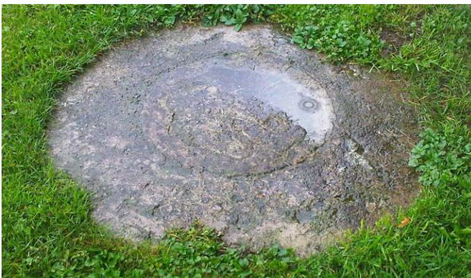
*A dug well. The well cap is located close to the ground and the well is prone to contamination. Know where your well is, how it is constructed and maintained, and how vulnerable it is to contamination.*
