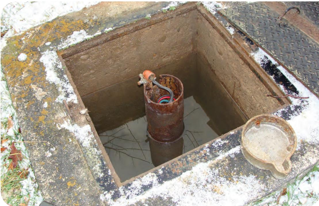
FIGURE 4: POTENTIAL SURFACE WATER CONTAMINATION
